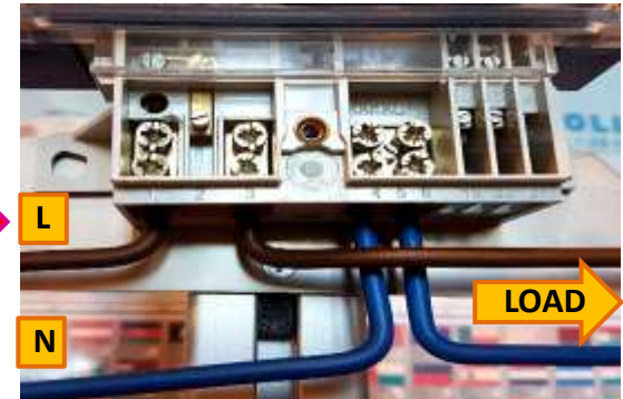
Wiring to meter terminals
