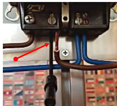
Connect instead „Cu” pin for safety cables
