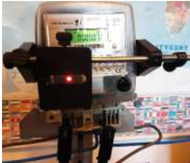
Assembly scanning head fix to see LED in hole
