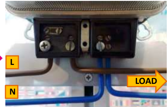
Wiring to meter terminals
