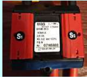
Typical current transformer CT in metering installation
